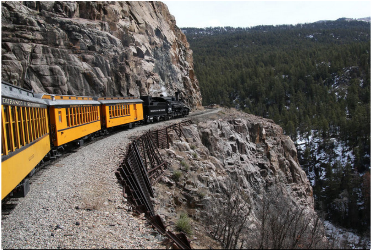
HIGH LINE CURVES – Rounding the sharp curves on the High Line north of Rockwood. The partially frozen Animas River is seen 400 feet below.
